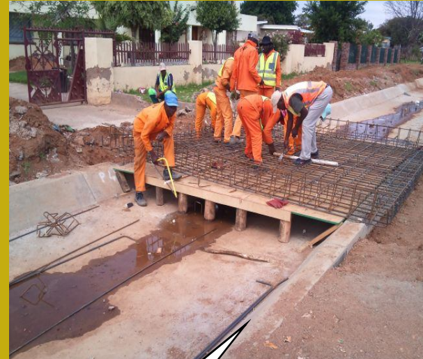
Reinforcing of access slabs
