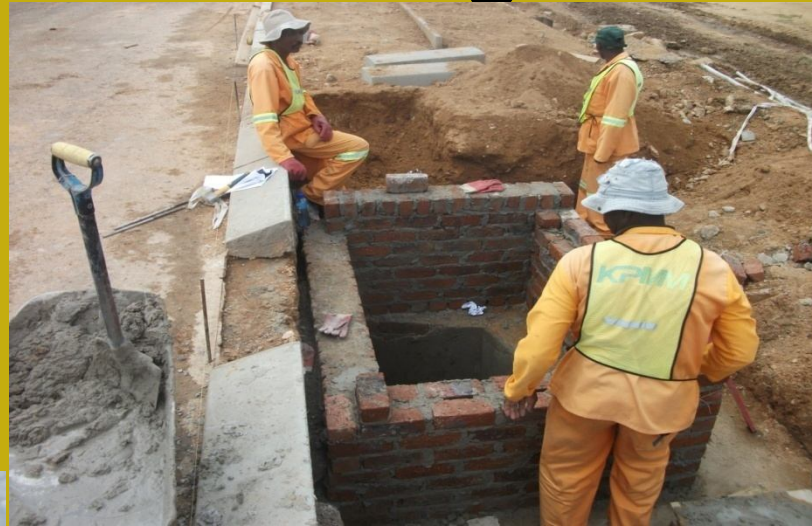
Constructing storm water junction boxes.
