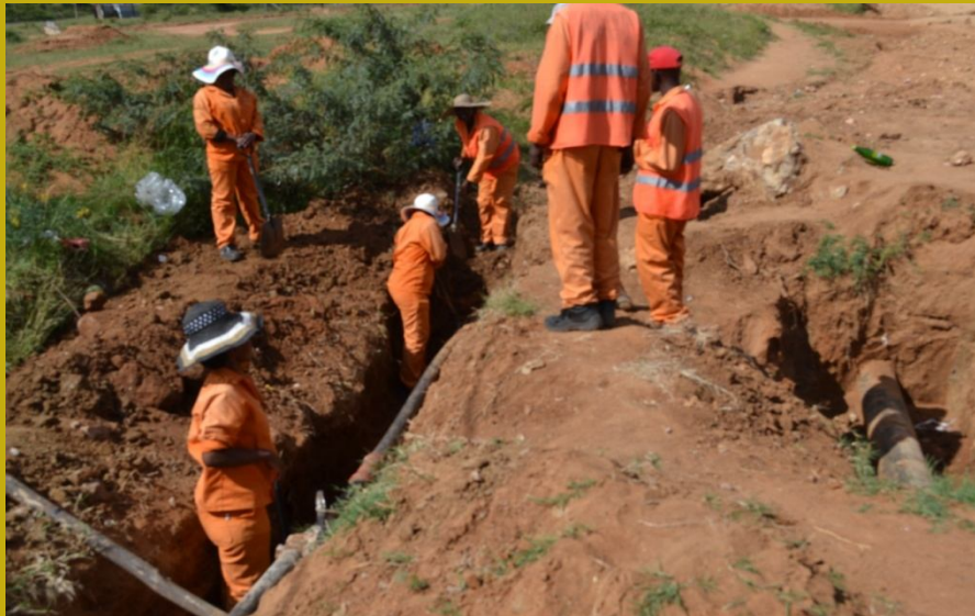
Pipe Relocation Excavation
