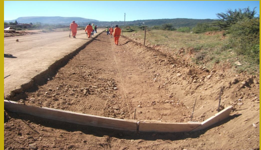
Concrete Drains Excavations
