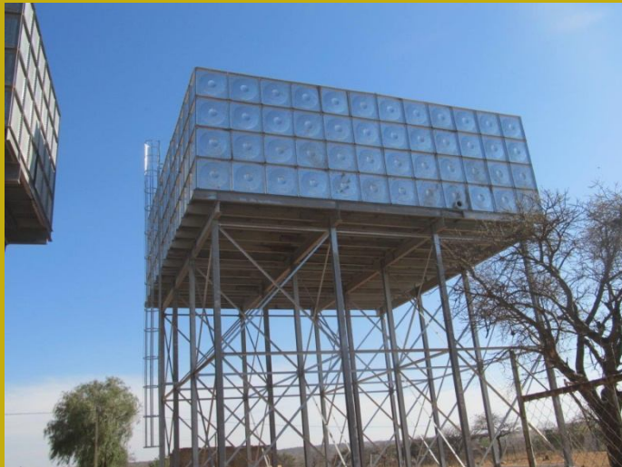
Completed tank with service pipe work
