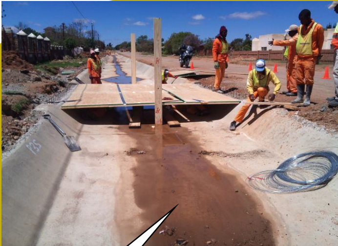
Shuttering of access slab
