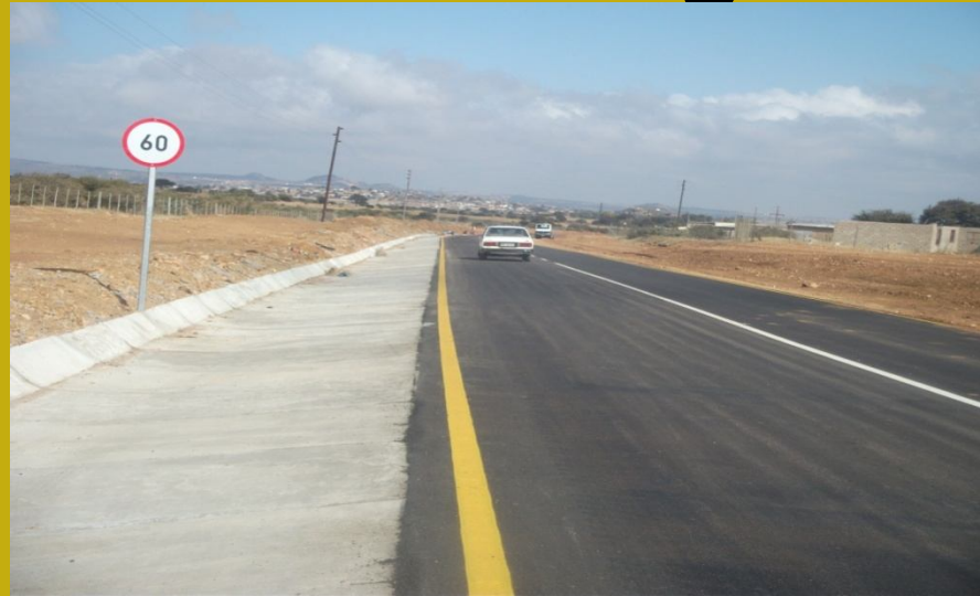
Complete Road with concrete Drains
