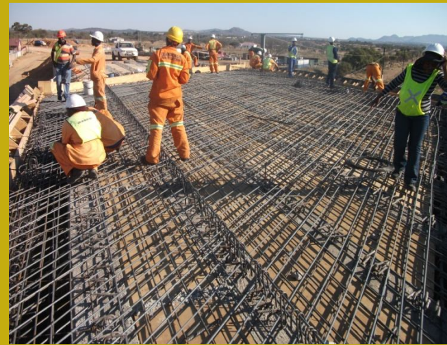
Local labourers fixing reinforcement on Bridge Deck
