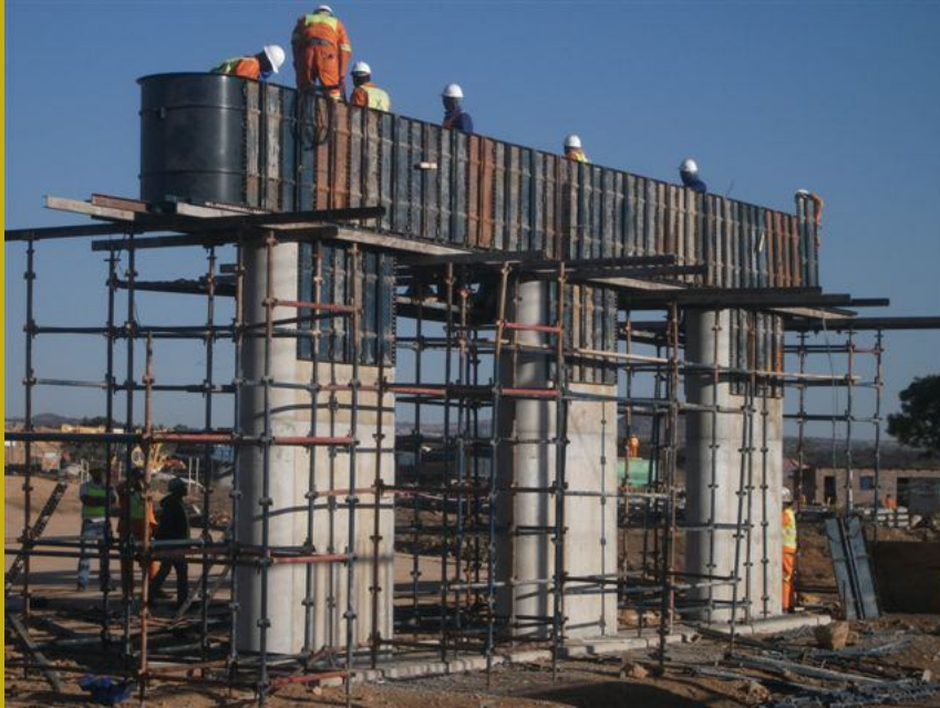
Local labourers fixing reinforcement on Bridge Deck
