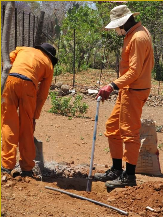
View of a stand pipe being installed.
