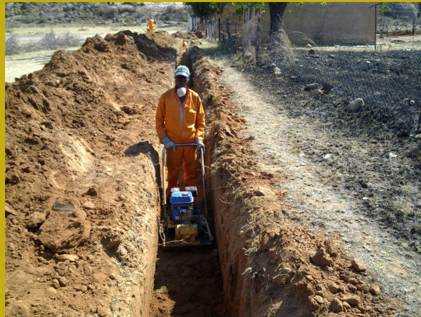
Compaction of backfilling
