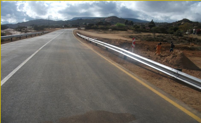
Guardrails Installed Using Labour
