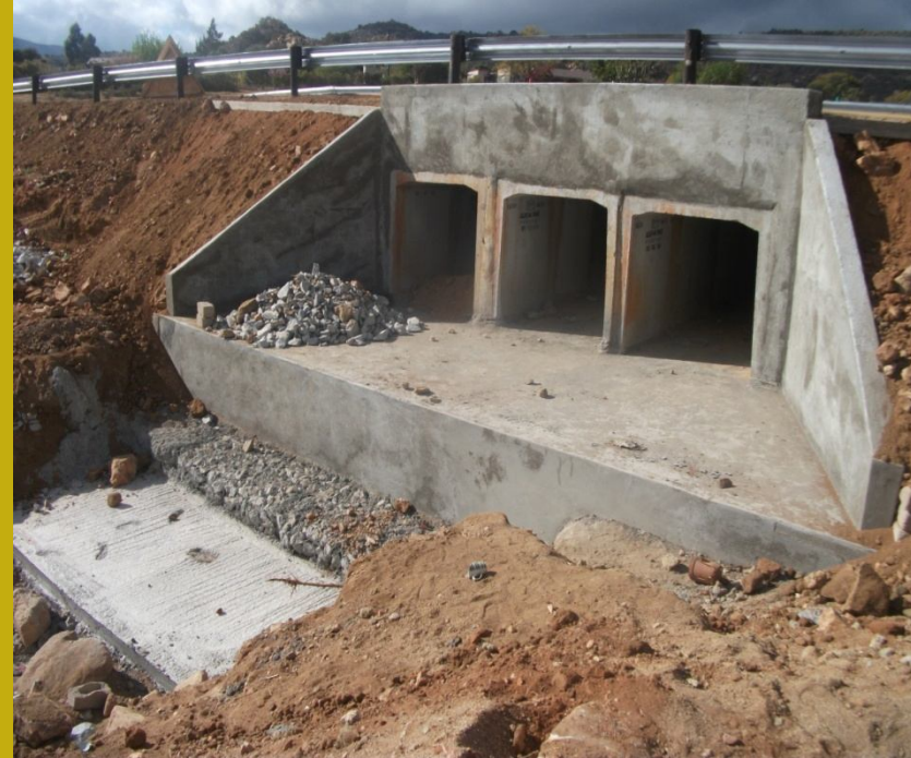
Complete Wing Walls Built Using Labour Intensive Method
