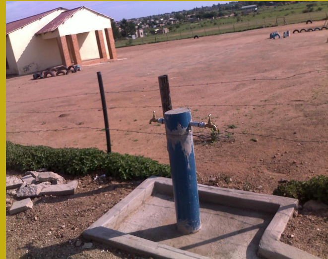
Completed standpipe
