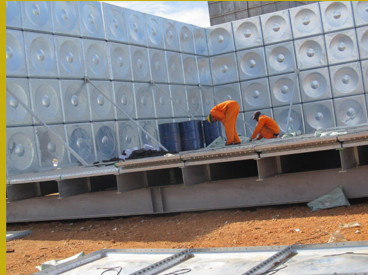
Reservoir panels being assembled
